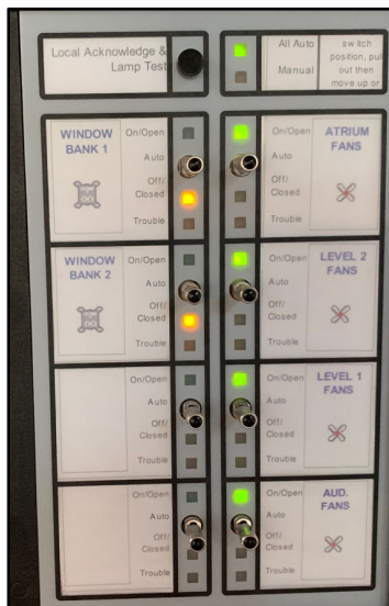
Smoke Control Override Panel
