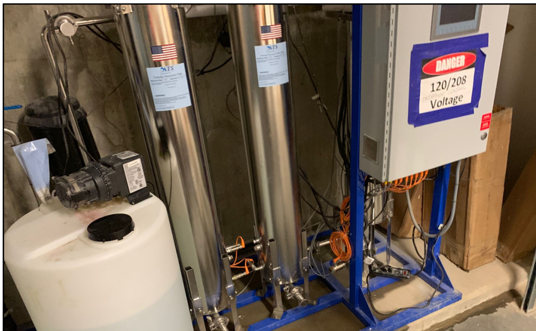
Potable Water Filtration Skid
