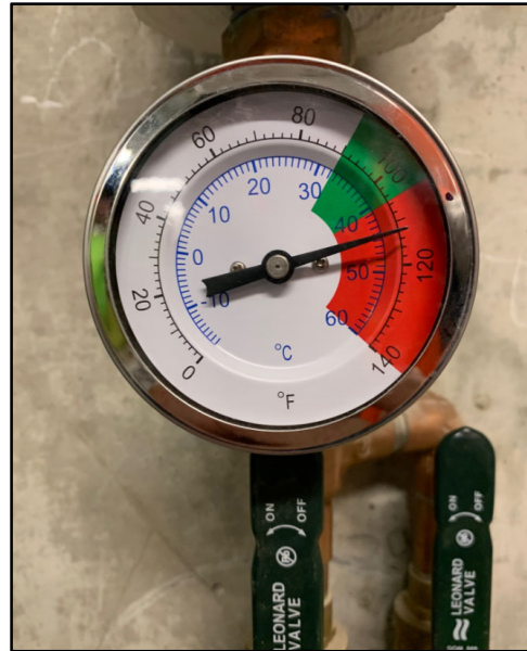
View of TMV Temp Gauge
