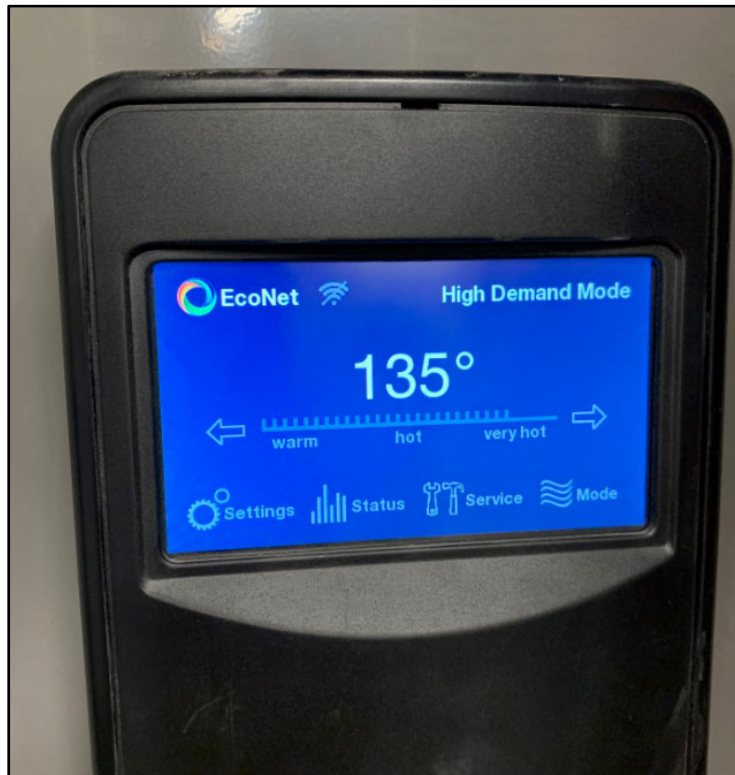
View of Water Heater Control Panel
