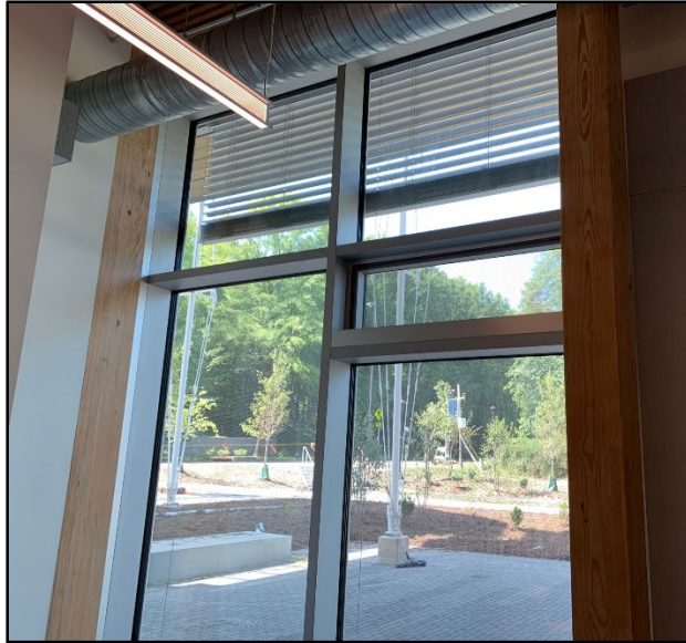
Typical Automated Blind Location
