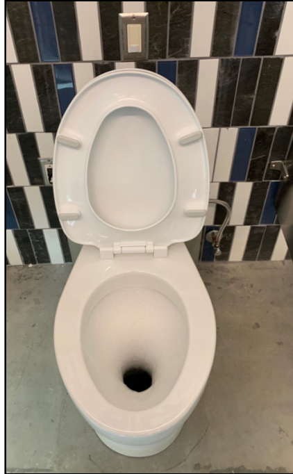
Kendeda Building Composting Toilet
